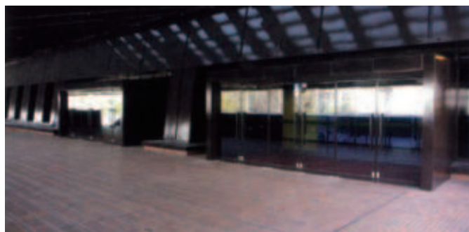
2階入口 Entrance 2nd floor
